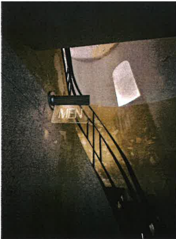
Stairs to Second Floor 2023
